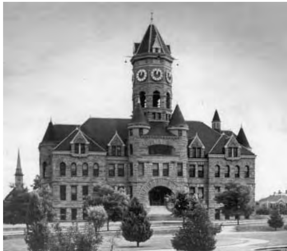
Thurston County Courthouse The state purchased the courthouse in 1901 and was used by the legislature from 1905 to 1928. The building, which is located at Legion and Washington St., now houses the offices of the Superintendent of Public Instruction.
