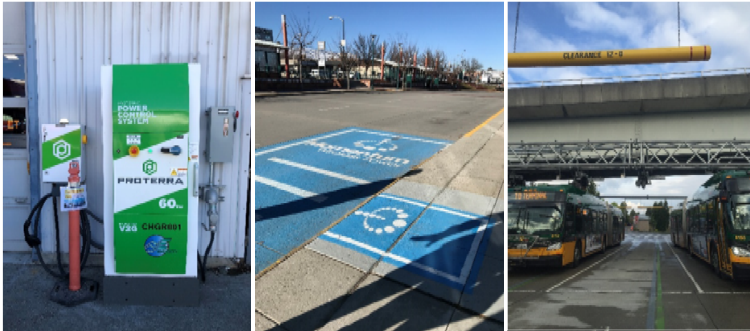
Left to right: Plug-in charger at Everett Transit, wireless charger at Link Transit, and KCM inverted pantograph charger at Eastgate Park-and-Ride
