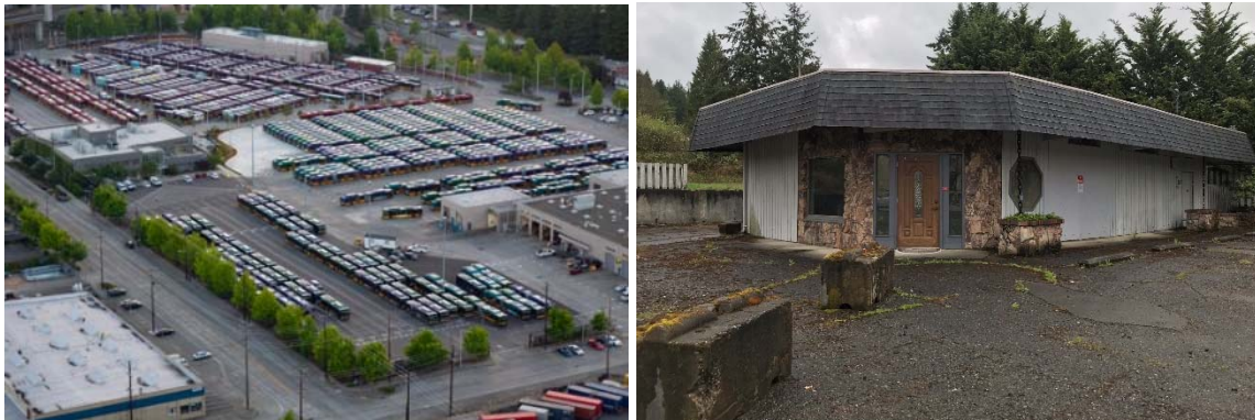
Left to right: King County Metro’s overcrowded Central/Atlantic Base; Twin Transit’s property for a potential small transfer center.
