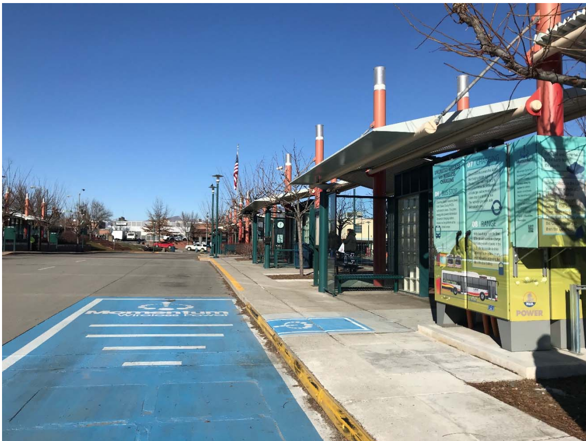
Figure 6-7 Link Transit’s Wireless Charging Zone at Columbia Station
