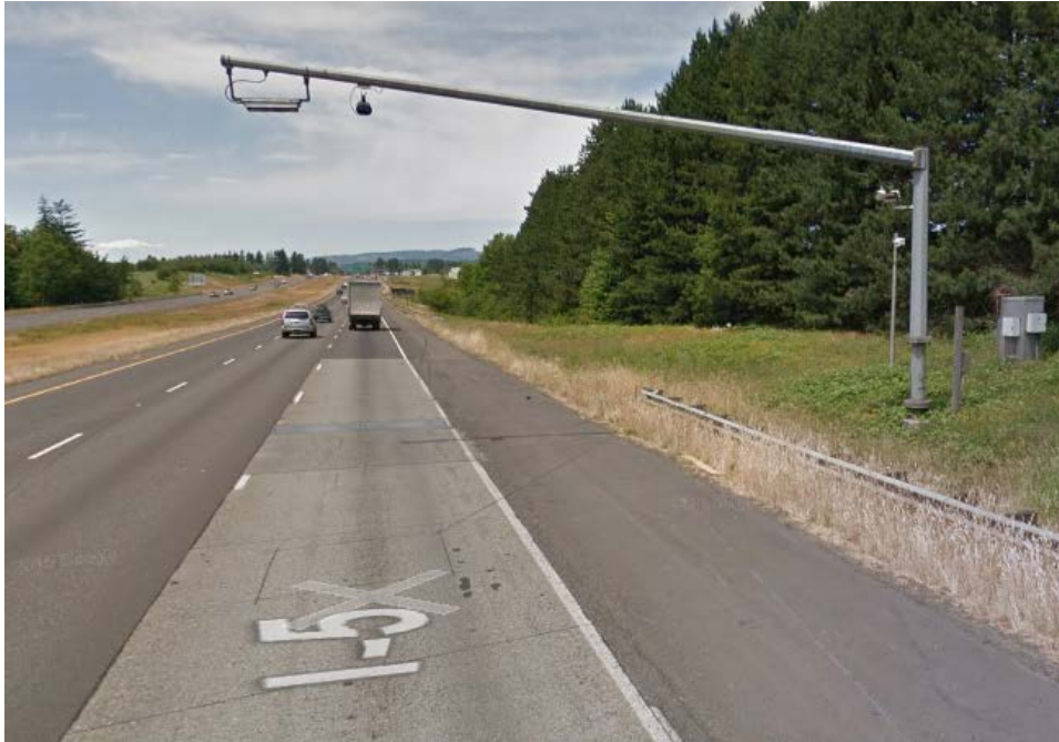
Figure E.3 Gantry Arm and WIM Pavement Segment Approaching Ridgefield POE
