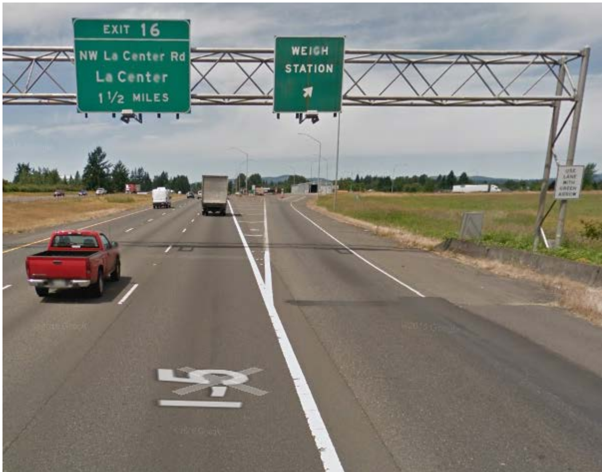
Figure E.7 Exit Ramp to Ridgefield POE
