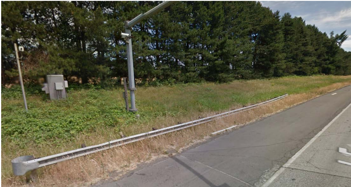
Figure E.4 Back of Gantry Arm, Approaching Ridgefield POE
