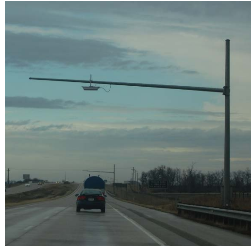
Transponder Readers (shown above) are one type of Electronic Screening
