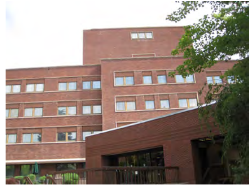
YVS Main Building
